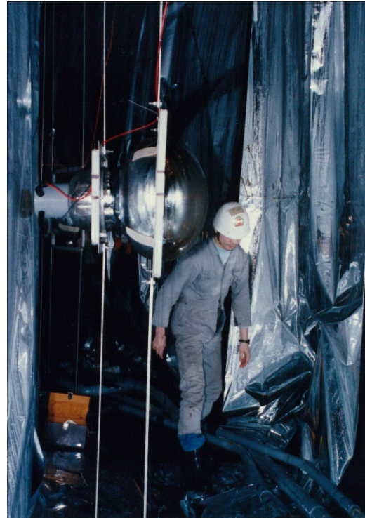
Side and bottom outer detector construction
