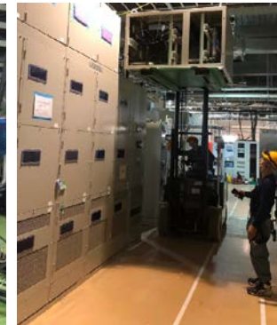
PS Upgrade work for RF Cavity
